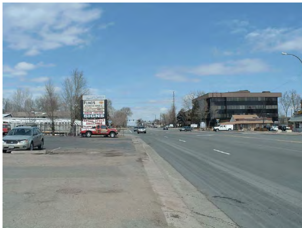
4. North View of Wadsworth Boulevard
