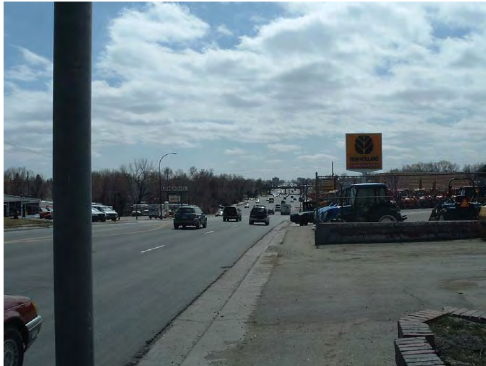
3. Wadsworth Boulevard South Bound Lanes
